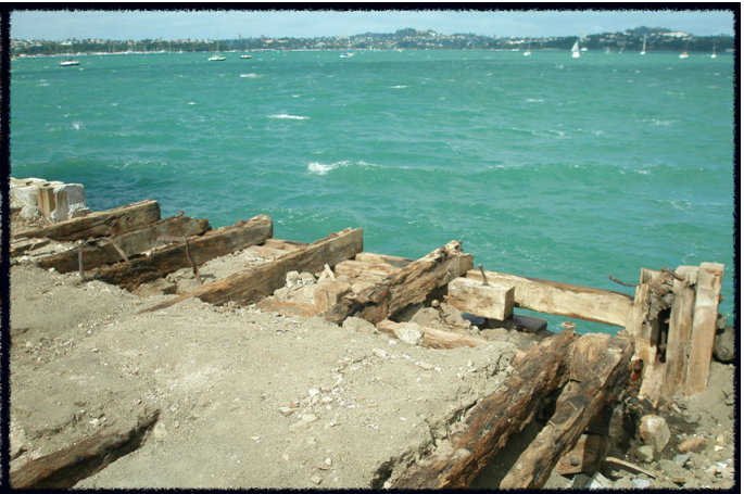
March 2010. The original pier head is exposed, studied and documented. This pier existed prior to the land reclamation which formed most of the present-day site. The sea wall originally reached the cliff face on the East of the site and to the modern-day administrative block, to the West.
