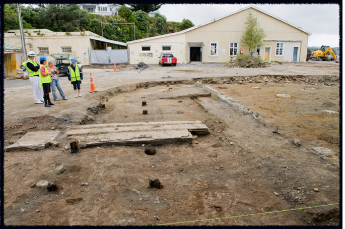
October 2009. Excavations revealed the rail lines from the 19th Century submarine mining station. Sea mines were transported around the site and hooked onto electronic cables before they were strung across the harbour to Bastion Point.
