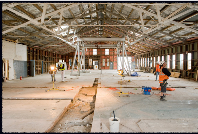
November 2009. The framing and exteriors of the buildings are preserved, while the interiors are gutted and fitted with new floors, walls and ceilings to provide temperature and humidity controlled spaces for the exhibition.
